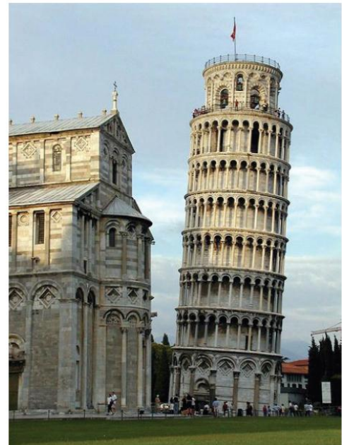
The Leaning Tower of Pisa, Italy. This is possibly the most famous example of "failed foundations".
